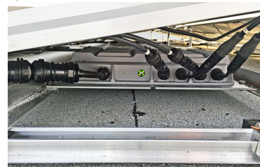
HiQ TrueString mounted under the array
